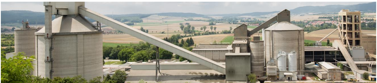
Dyckerhoff cement plant Göllheim: the raw meal from this plant is being investigated for its usability in the Indirectly Heated Carbonate Looping process. Source: Dyckerhoff.
